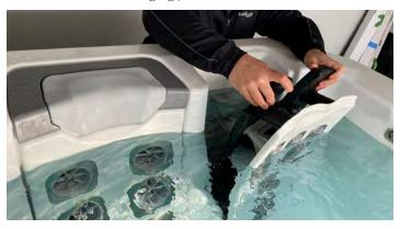
**Step 3:** Remove the Simplicty filter holder. Reach down into the jet pod and grab the handle, push toward the middle of the spa and lift up to remove from the housing. Place holder on a flat
