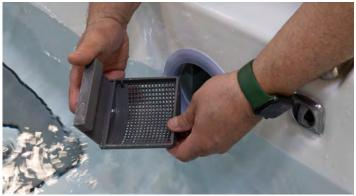
**Step 5:** Return baskets to their original installed location inside the filter intake fixture and replace grate assembly by snapping into place.
