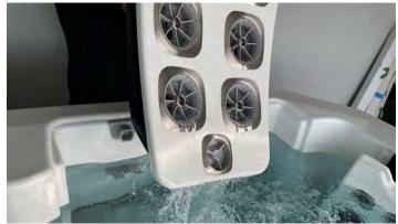
**Step 5:** Lower the manifold of the new JetPak carefully as to align the lower valve assembly and gasket into the bulkhead fitting. Apply pressure downward as you move the JetPak manifold until the manifold is secured in the wall clip assembly. **Step 6:** Replace the Snap-Cap and head rest over the JetPak and press down firmly to snap into place.
