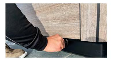
**NOTE:** Drain is fully extended at approximately 2 inches (5 centimeters).
