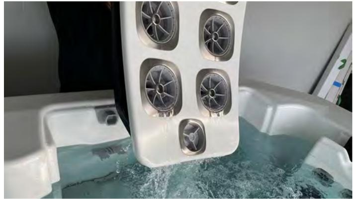
**Step 5:** Lower the manifold of the new JetPak carefully as to align the lower valve assembly and gasket into the bulkhead fitting. Apply pressure downward as you move the JetPak manifold until the manifold is secured in the wall clip assembly.
