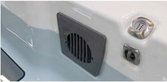
**Step 2:** Remove the filter grate by pressing both of the locking tabs on each side outward while pulling the grate away from the intake fixture and spa wall. Set grate aside.
