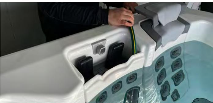
**Step 3:** Fill to the water level indicator or the mid point of the filter intake grate and proceed to start up procedure.
