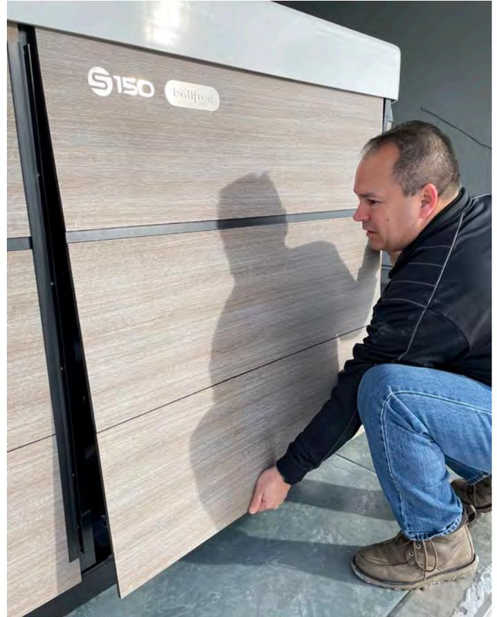
**Step 2:** Replace trim strips by snapping each strip carefully into the trim channel.
